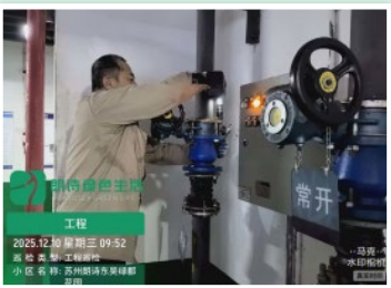
管件法蘭螺栓緊固 Tightening of Pipe Flange Bolts
